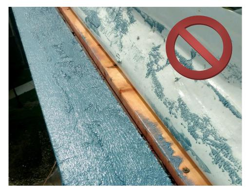
Also make sure that we use wood with no large or loose knots, as these are unacceptable deflects in the wood which could dislodge over time.
